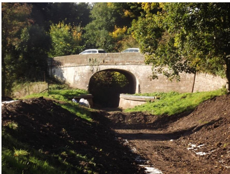
Figure 16 The Skew Bridge
