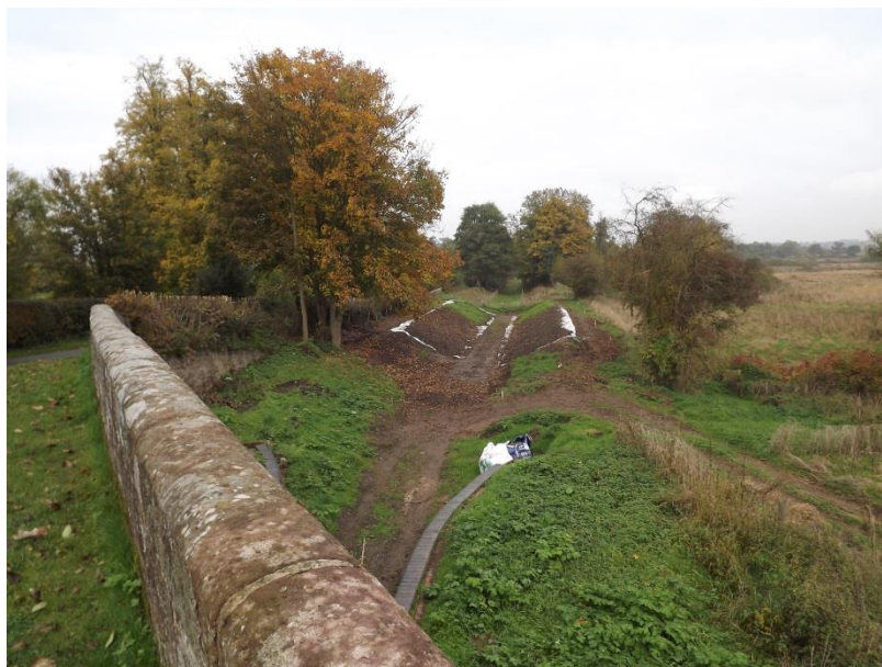
Figure 45 View of branch canal excavation from Skew Bridge
