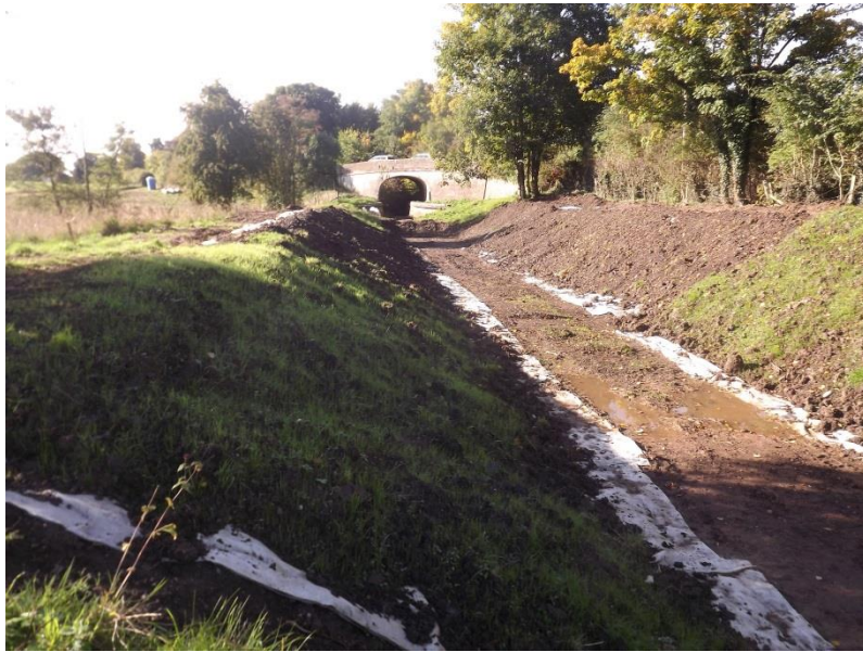
Figure 44 Recent excavation of the Newport Branch Canal looking towards Skew Bridge
