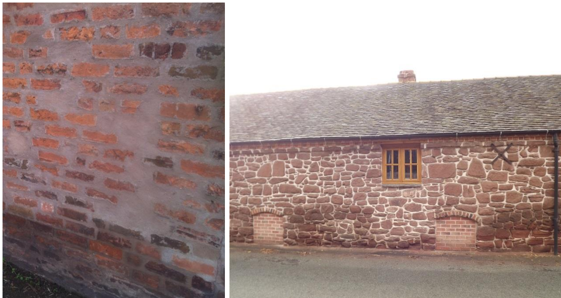
Figure 40 The use of cementitious mortar can both mask and detract from historic masonry
