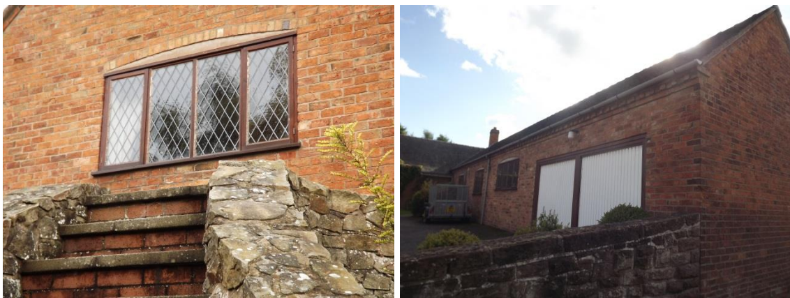
Figure 42 Modern windows and doors can have an adverse effect on historic character
