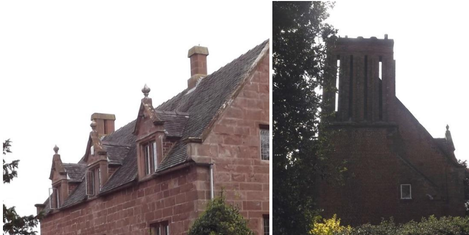
Figure 8 Roof dormers and finials at Forton House and chimney stacks to Forton Hall
