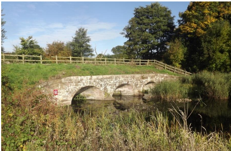
Figure 15 The Forton Canal Aqueduct
