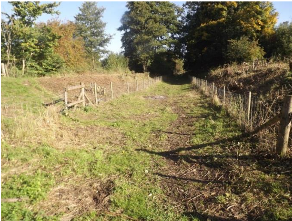
Figure 34 Site of the former branch canal to the north of the Skew Bridge
